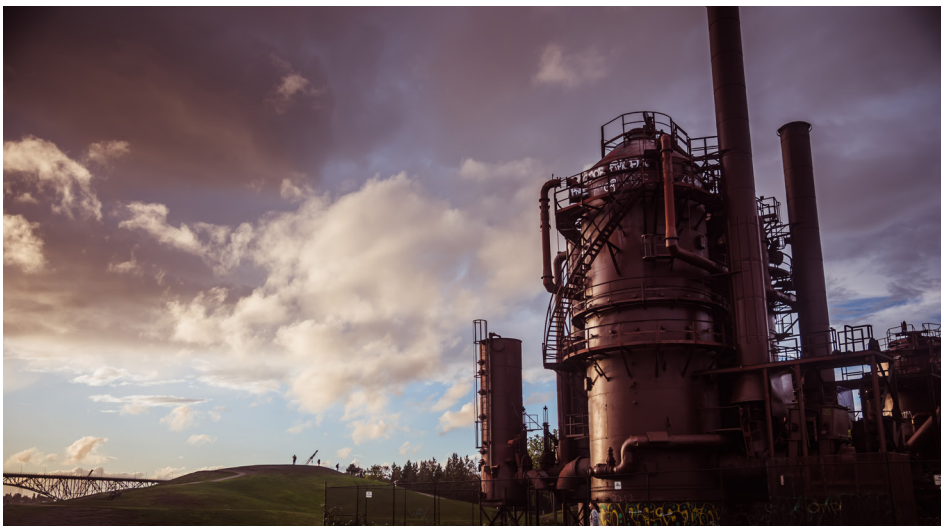
Natural Gas Energy
